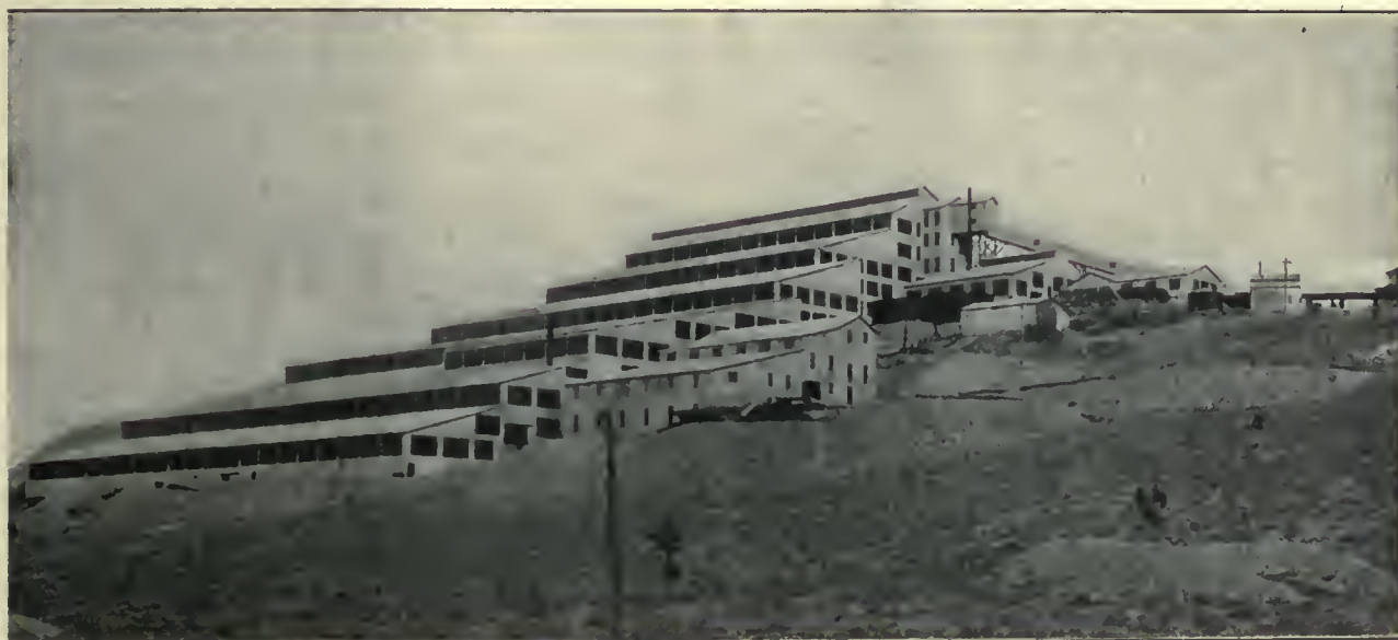
GOLDFIELD CONSOLIDATED MILL.
